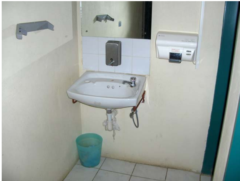
Figure 22: Clean hand washing bay
