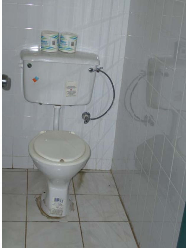
Figure 23: Clean washroom facility
