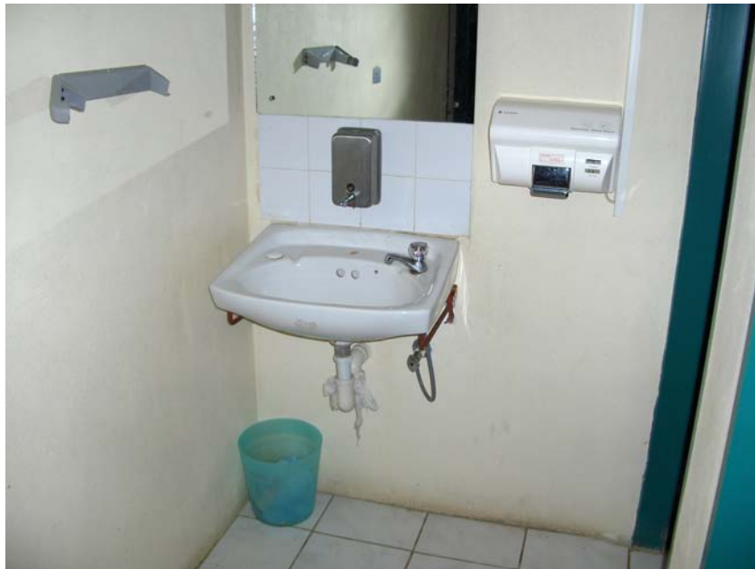
Figure 22: Clean hand washing bay
