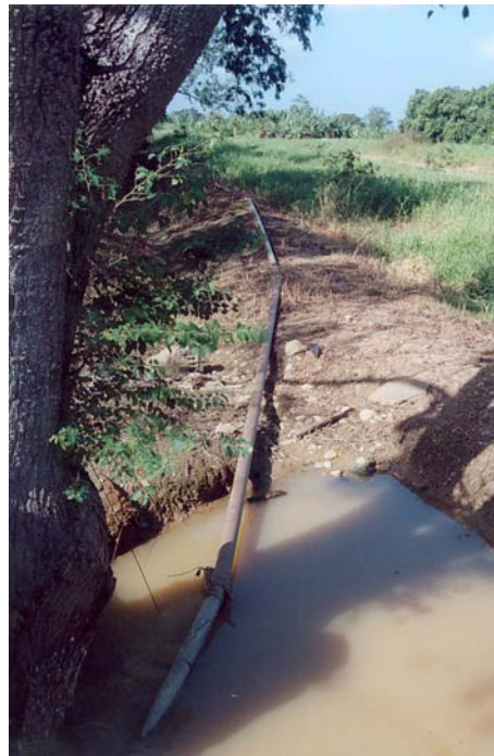
Figure 10: Galvanise conduit pumping polluted water into production fields
