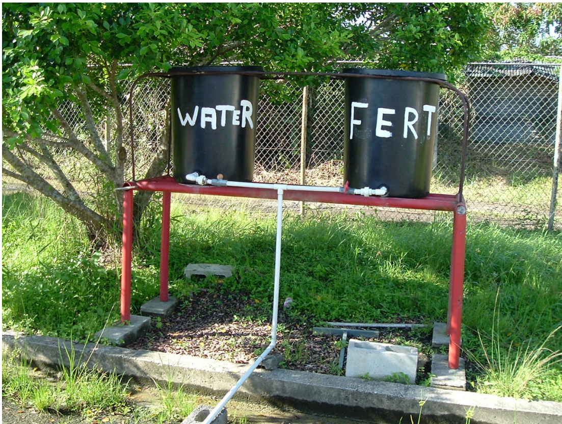
Figure 5: Separate tanks used for irrigation and fertigation are clearly marked.
