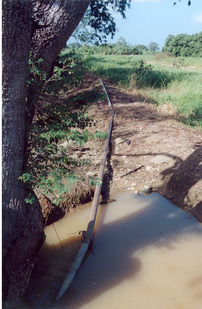
Figure 4: Galvanise conduit pumping polluted water into production fields
